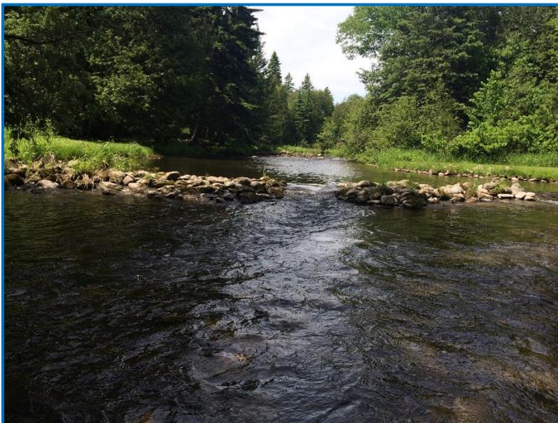
**Photograph 9. Breached man made dam within West Credit River study area, looking upstream**
